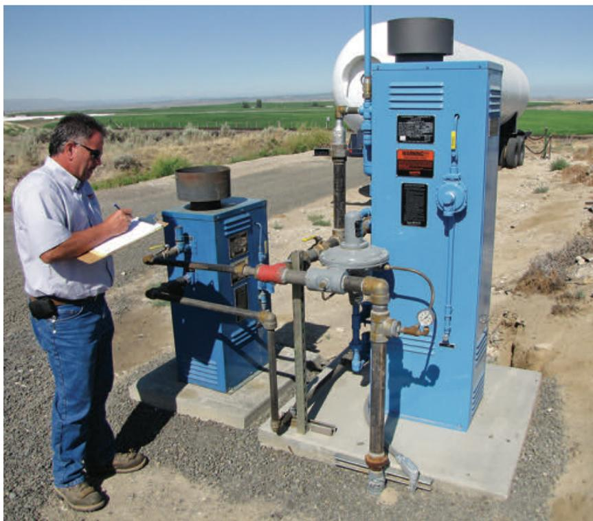
**A portable (“Port-A-Pack”) 18,000-gal. trailer is connected to two vaporizers for a mint processing plant. “The boilers and mint dryers use so many Btus that it requires the vaporizers to help vaporize the liquid propane to supply the high demand,” said Darcy Start of All American Propane.**
